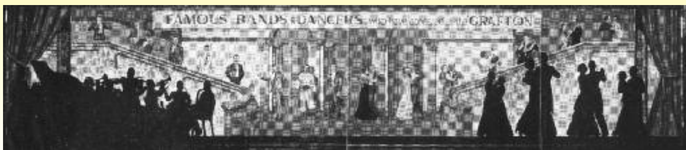
The painting of the stairs of the Grafton Rooms, Liverpool
